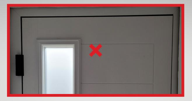
4) The slight bending in of the top frame pushes the sash towards the lock side creating uneven air gaps, resist the temptation to adjust the hinge. Instead simply **insert a packer behind where your top fixing** will go.
